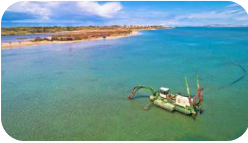
Figure 19: Dredging and sand mining damage seagrass by removing or burying it and clouding the water, blocking the sunlight these plants need to survive.
